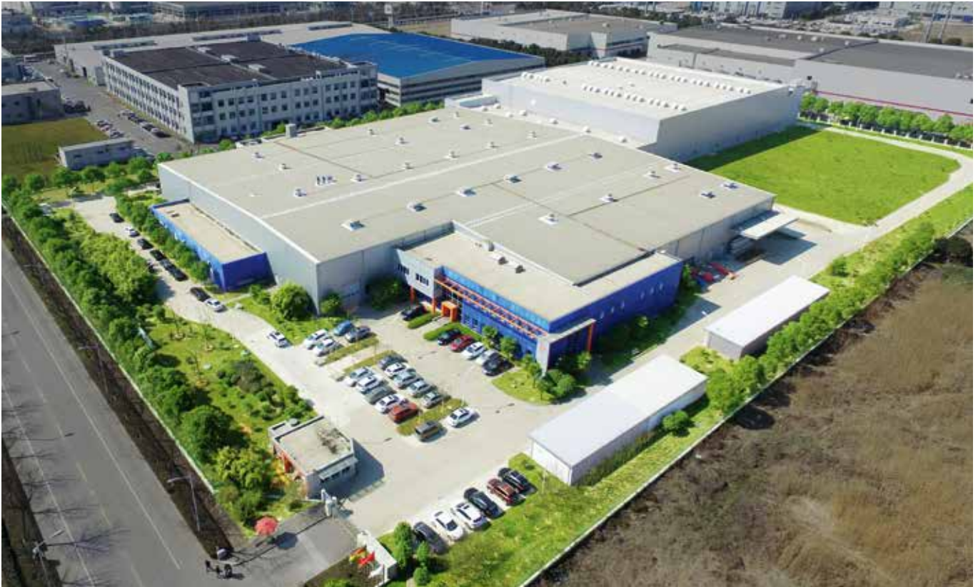
Factory in Suzhou, China
