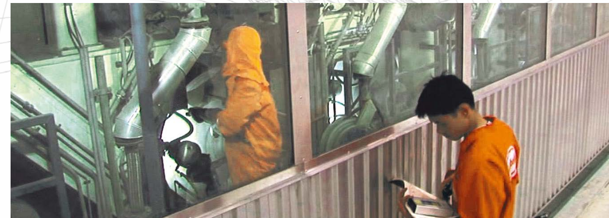
Fig. 5: Temperature measurement in the dryer hood
