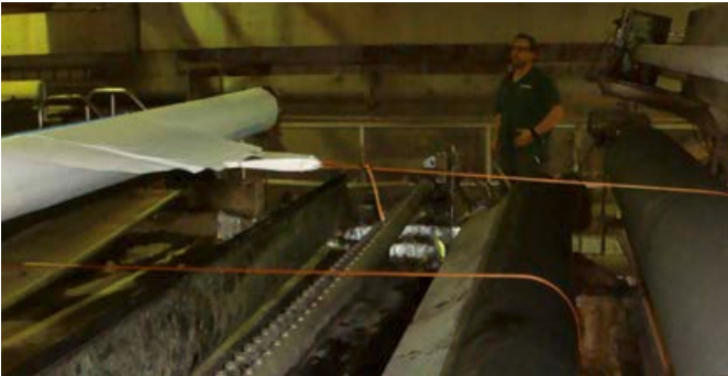
Photo 4: Ready for pulling in.
