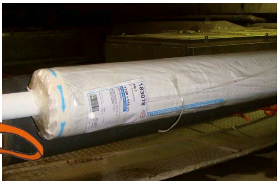
Photo 1: Atromaxx.Connect ( still in its' protective wrapping ) ready for installation.
